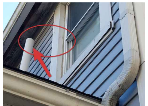
Plumbing vent too close to window.
